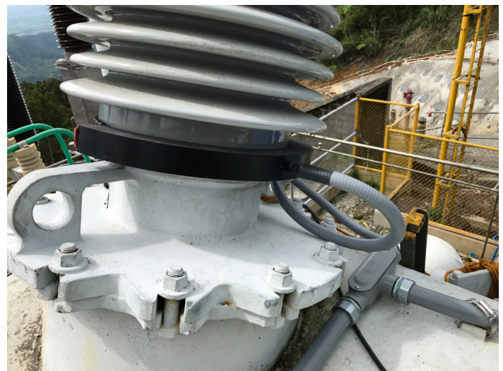
UHF Bushing Sensor Type B800
