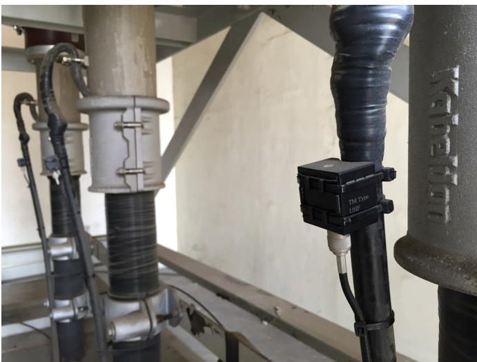
Cable Termination UHF Sensor Type TM
