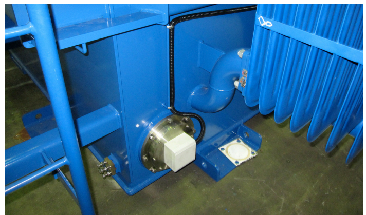
Transformer UHF Hatch Sensor Type T10
