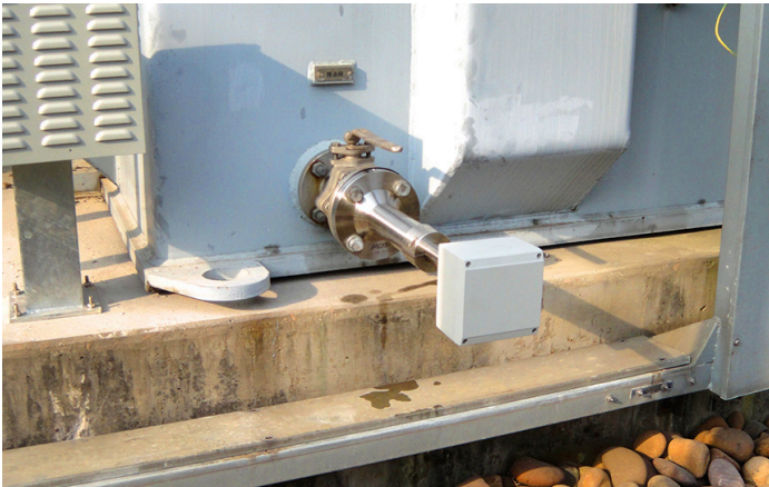
Drain Valve UHF Dn 50 Sensor
