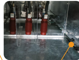
TEM Sensors on Switchgear
