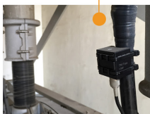
Cable Termination Sensor: TM
