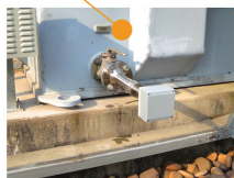
Tfr. Drain Valve Sensor
